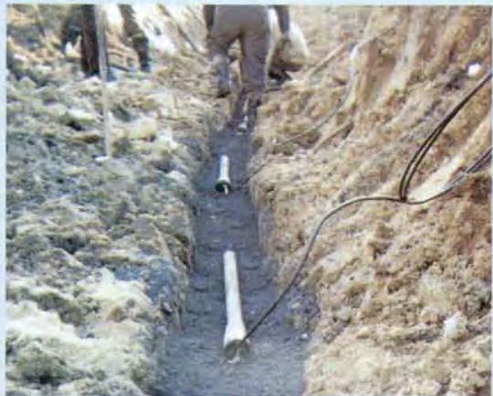
Standard Horizontal Groundbed installation utilising Silicon Iron anodes
