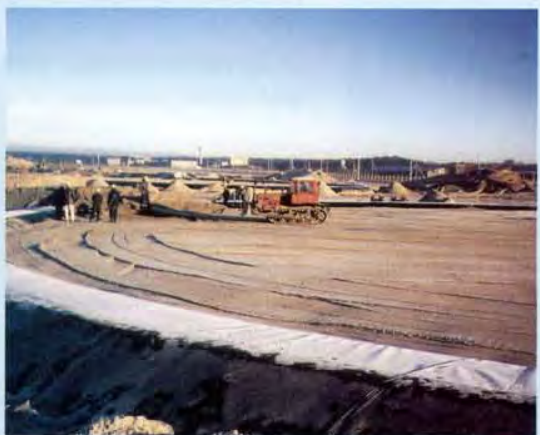
Tank base Cathodic Protection system installation
