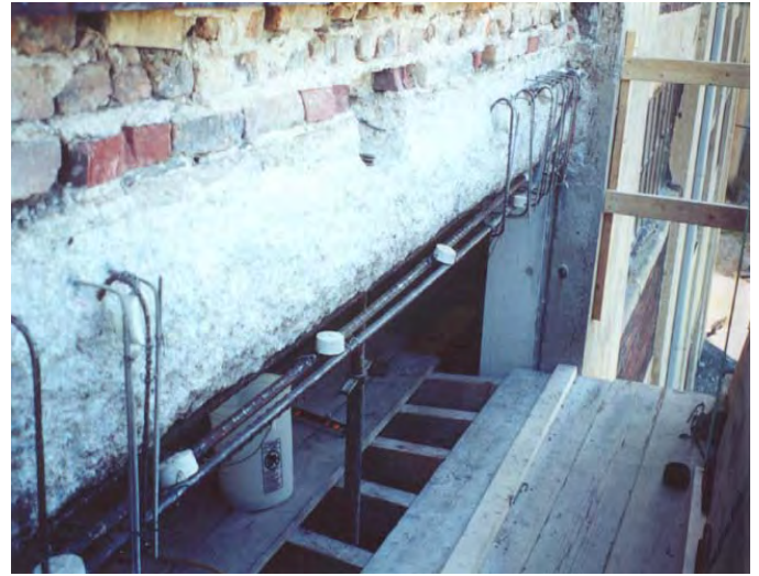
Figure 9. Installation of mortar enhanced zinc anodes in a concrete repair
