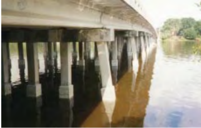
Figure IV. Integral pile jacket system on bridge piles in Florida.
