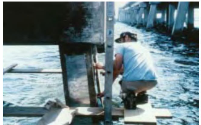
Figure VIII. Zinc adhesive anode being applied to a bridge pier in Florida.
