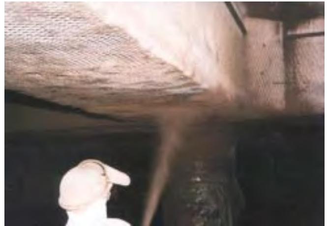
Figure III. Titanium anode mesh encapsulation with shotcrete, Hong Kong container berth.
