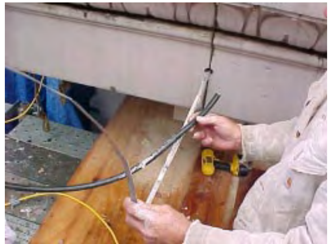
Figure 5. Discrete titanium anode installation in terra cotta cornice.
