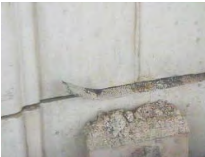
Figure 4. Titanium Ribbon Mesh installation in mortar joint.
